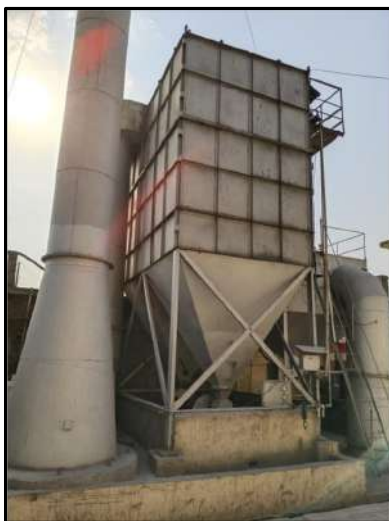
Photographs showing APCD & Stack
